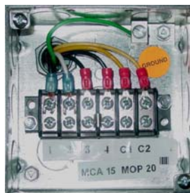
Figure 2.8. Atlas Field Wiring Box
