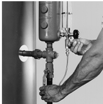
Blow down the water level control each morning by opening the control and water gauge blow-off valve.
