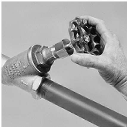
Blow down the boiler weekly. Shown here is blow down "Y" value.
