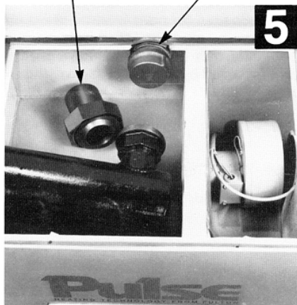
Disconnect Bleed Lines, Separate Gas Train From Gas Decoupler
